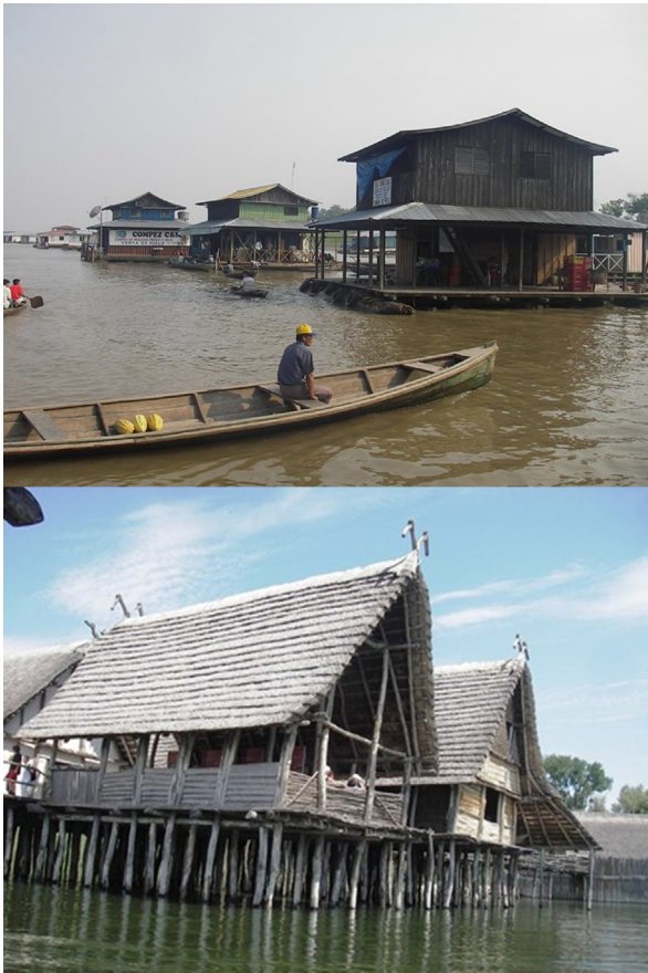
Fig. 4. Traditional architecture adapted to the rhythm of the waters. Above: floating house in Leticia, Amazonia Colombia; below: reconstruction of a neolithic stilt house, Unteruhldingen, Lake Constance, Germany.
